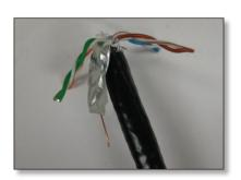
7. Place the wires in order as shown in the Cable Wiring Specification (T568B), ensuring they are as straight and compact as possible.
